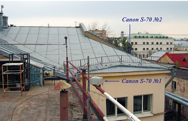
Fig. 3. Model of a stereo installation for determining the height of the lower cloud boundary on the roof of the IAP RAS.
